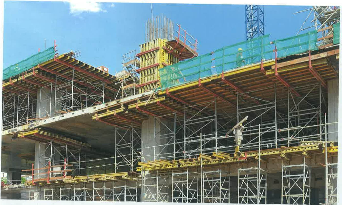
Large-area PD 8 slab tables with SRZ as main beams and VT 20 as cross beams combined with PERI ST 100 Stecking Tower.
