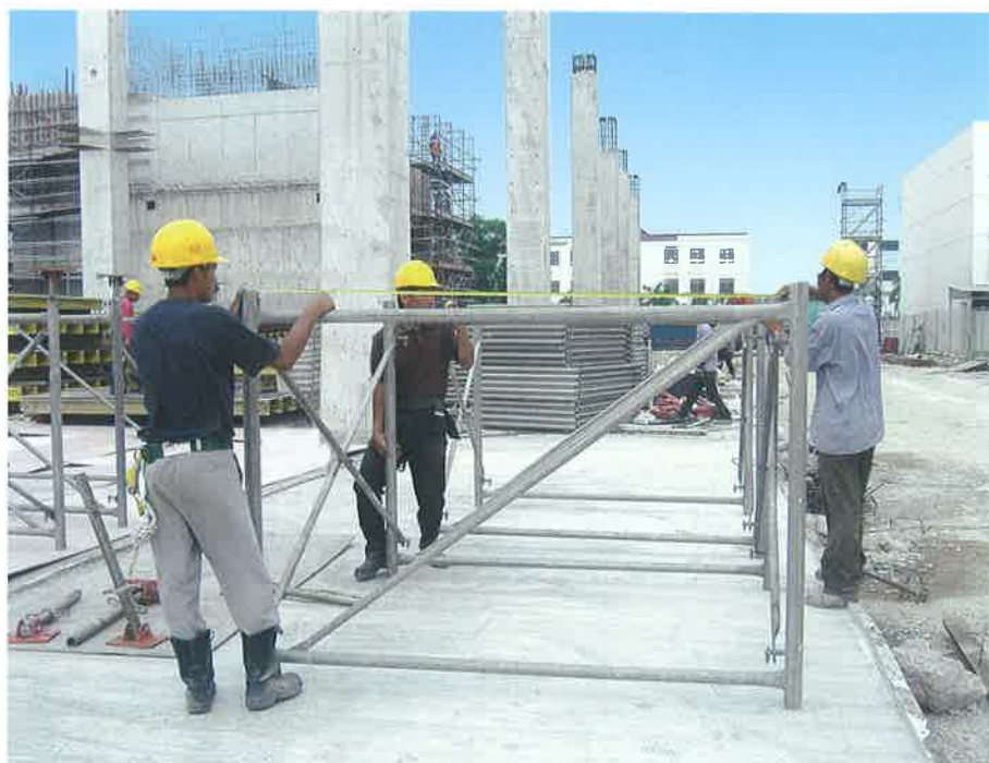
Basic assembly of the PD 8 slab table can be carried out manually.
