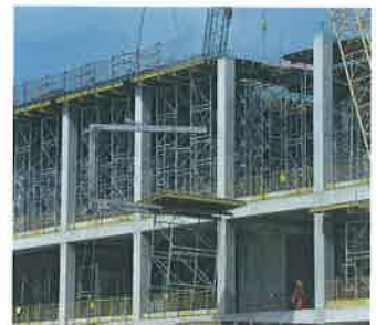
PD 8 slab tables moved with the Lifting Fork 1.75 t / 8.0 m.
