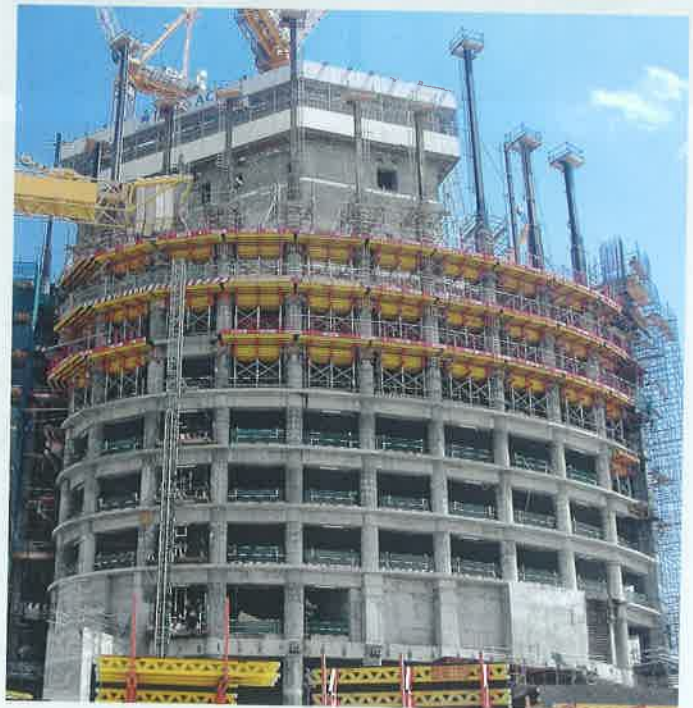
PD 8 table complete with guardrails for forming the edge beams of a high-rise building.
