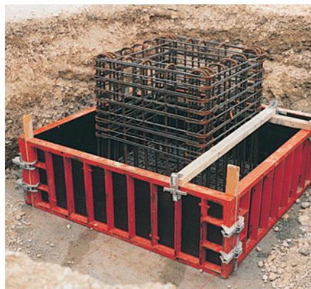
Panels being used on their side for foundations
