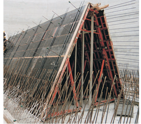
Trapezoidal tunnel with TRIO and SKS brace frame.
