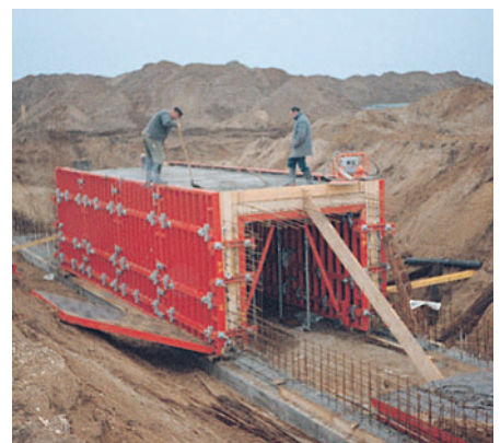
Rectangular tunnel with standard TRIO components.
