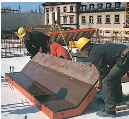
135° corner panel, fitted with large formlining sheets, being used in the construction of a Hotel.
