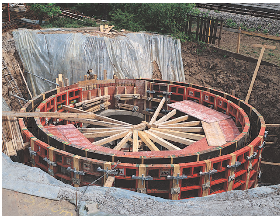
Sewage tank shuttered with TRIO TR 270 x 60 panels.
