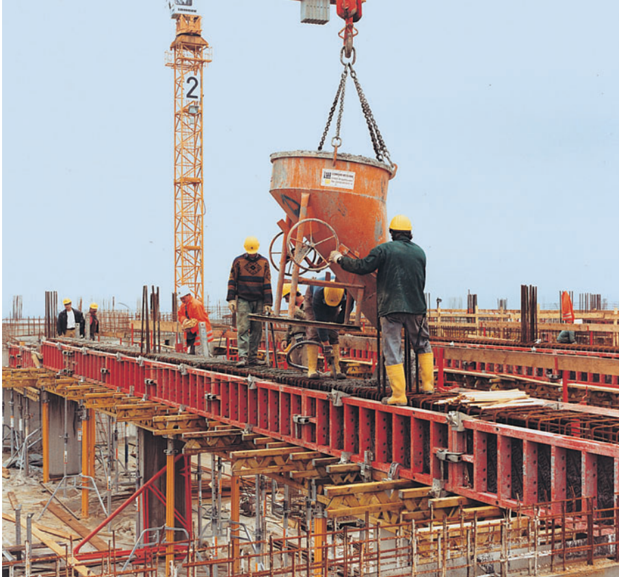
Small beams with TRIO. Supported with MULTIPROPS.
