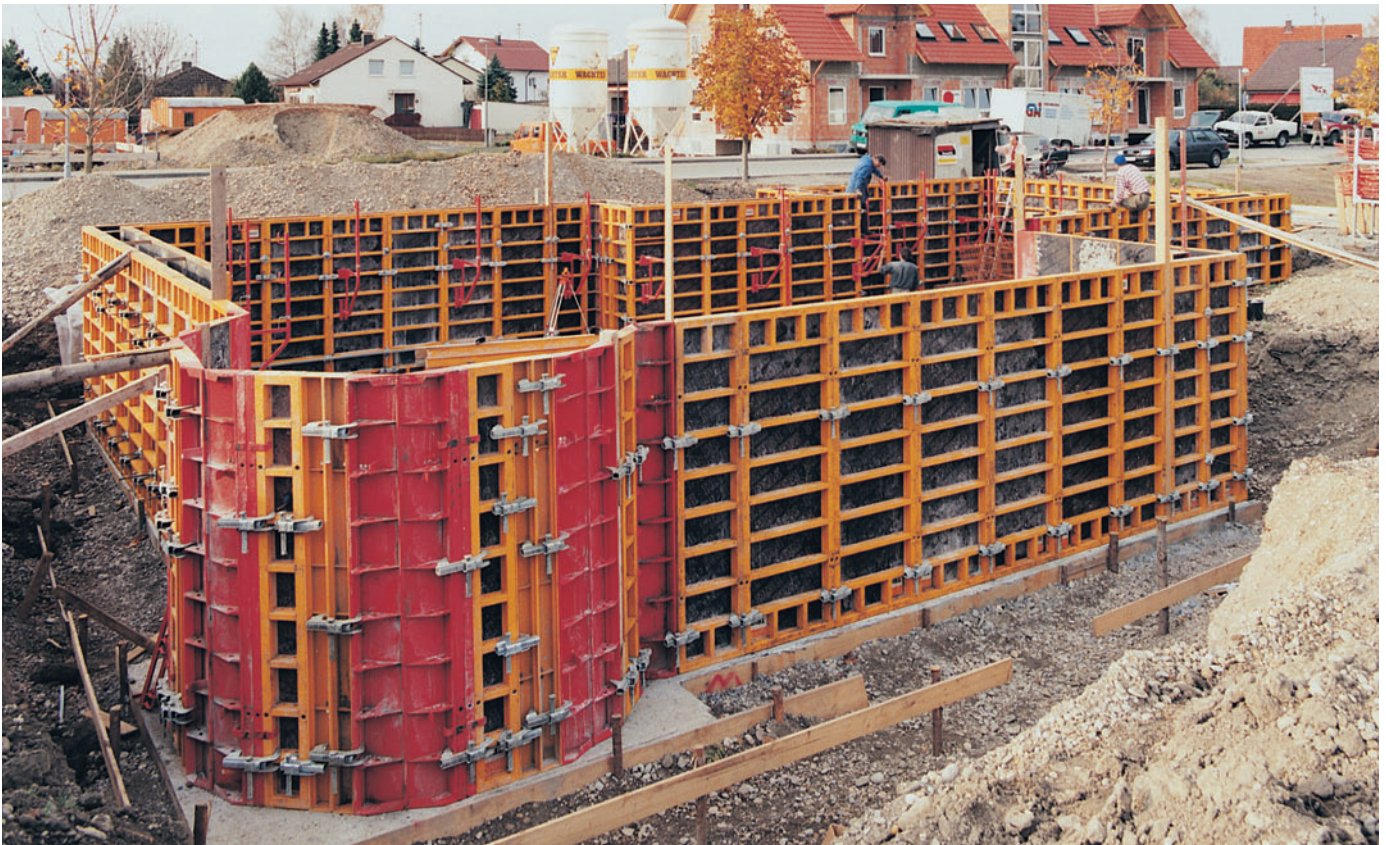
4 panel widths are available in heights of 270 and 900mm as TRIO-L.
