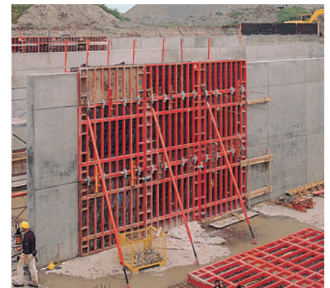
TRIO panels on their side and extended to a height of 6.0m
