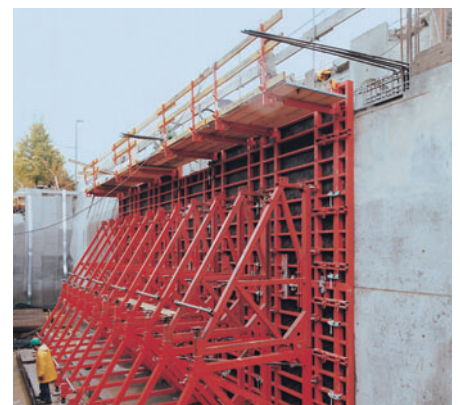
Single sided formwork
