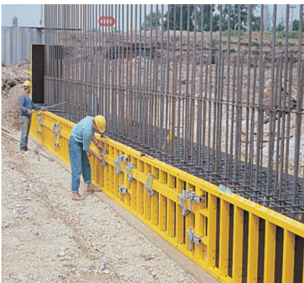
TRIO-L being used to shutter foundations.
