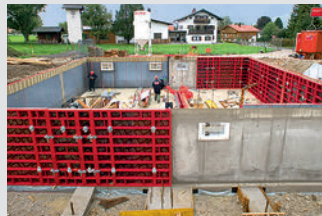
Wall Formwork
