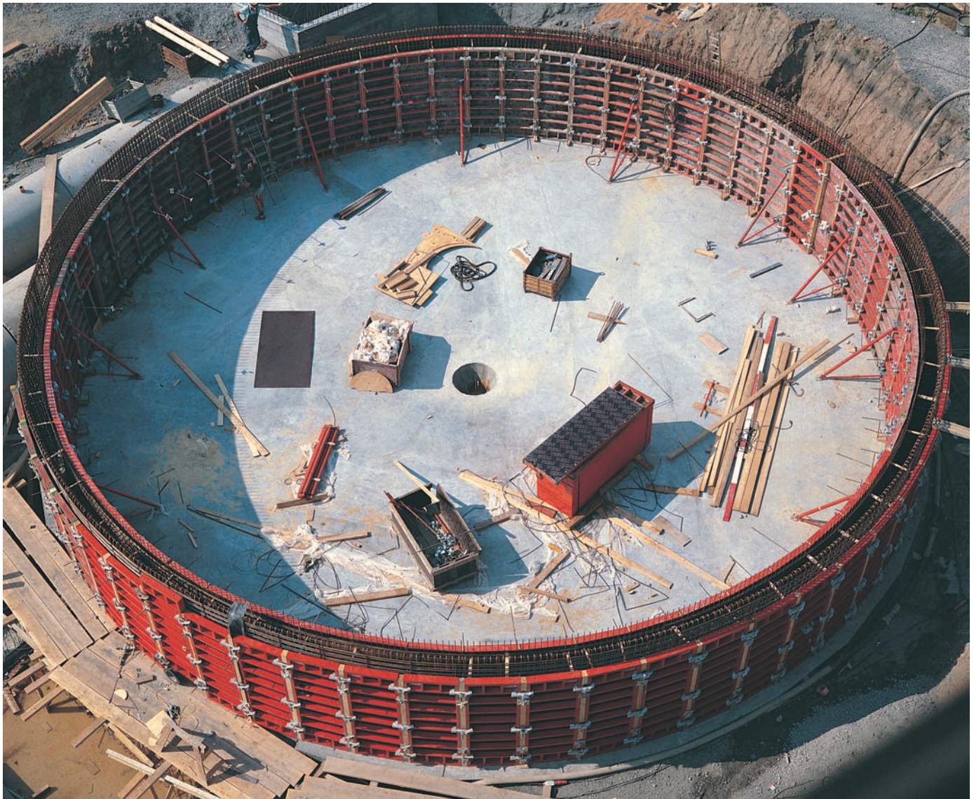
Stormwater tank with a diameter of about 18m, shuttered with TRIO TR 270 x 90 panels.
