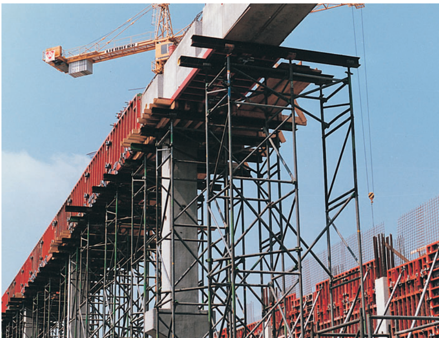
Heavy beams with TRIO.
