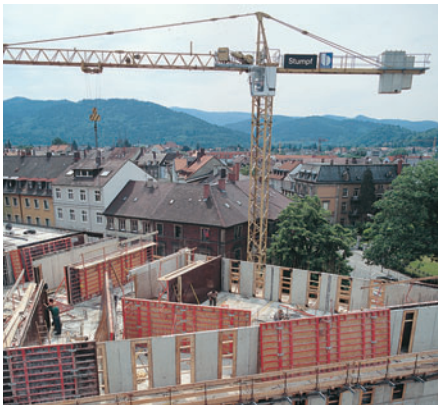
Panel units up to 9m wide and 2.70m high fitted with large formlining sheets.
