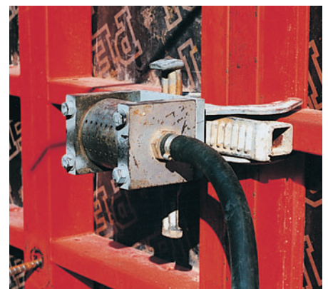
Connection of external vibrators
