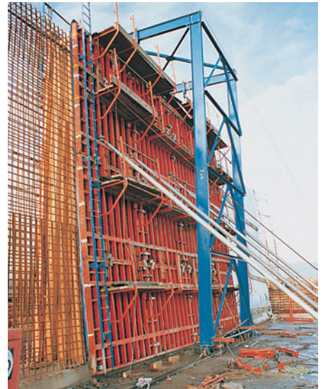
Complete TRIO unit 8.40m high. Inside and outside formwork hung from a portal frame traveller.
